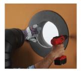
4- Then, from outside the building, slide a short chimney length (attached to the tee) through the wall thimble. The chimney must extend at least 3 inches into the living space where it attaches to the stove pipe.
